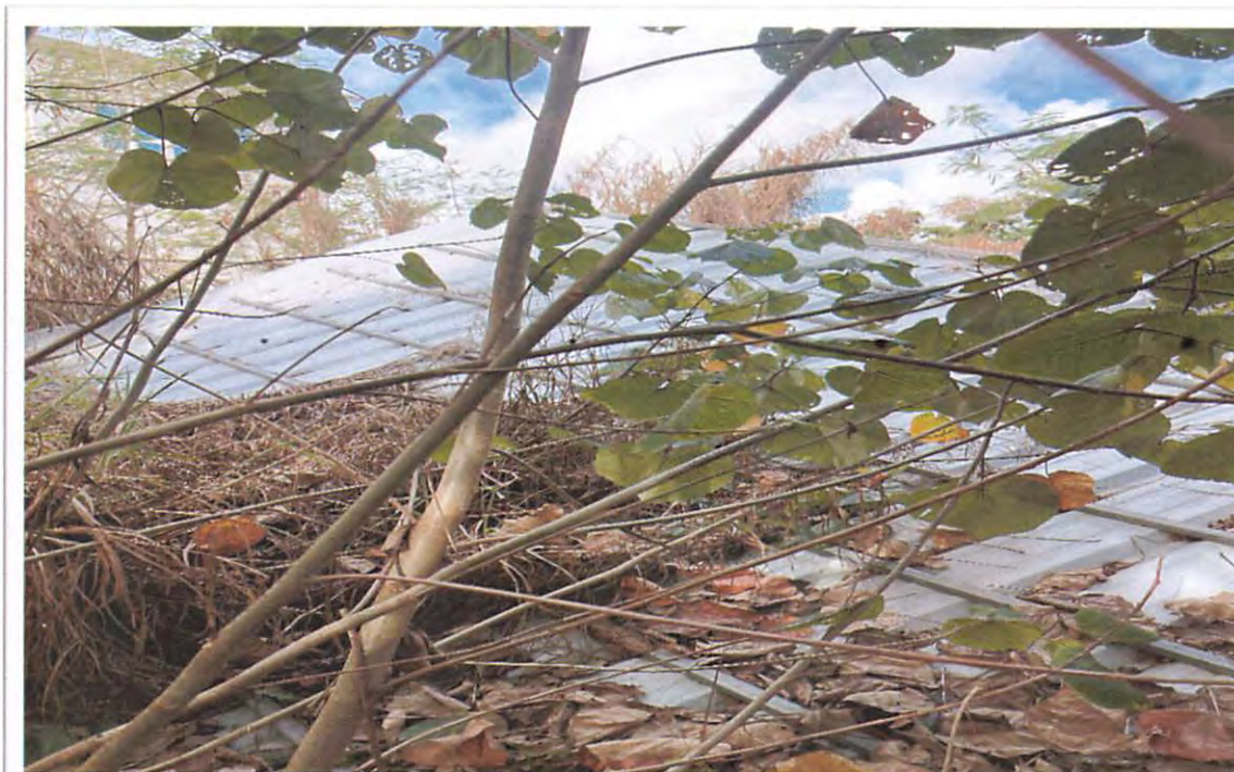
Photo 16. Metal Roof in in southwest region of the site.
